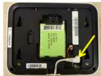
DISCONNECT POWER CABLE
